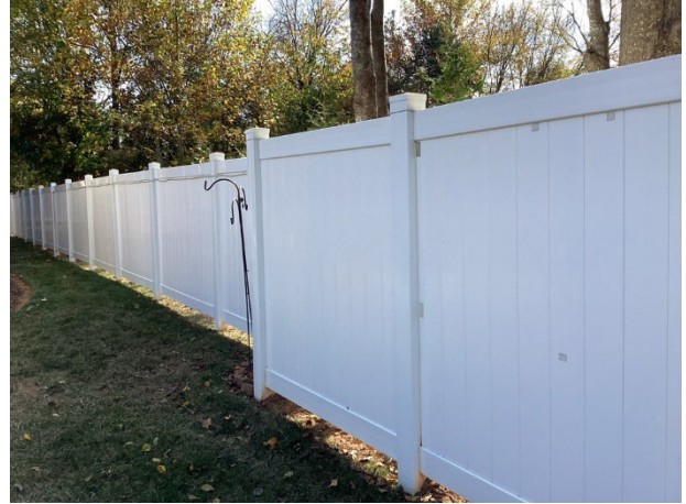
Vinyl fence at perimeter
