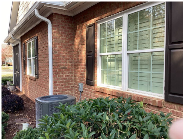
Masonry walls overview
