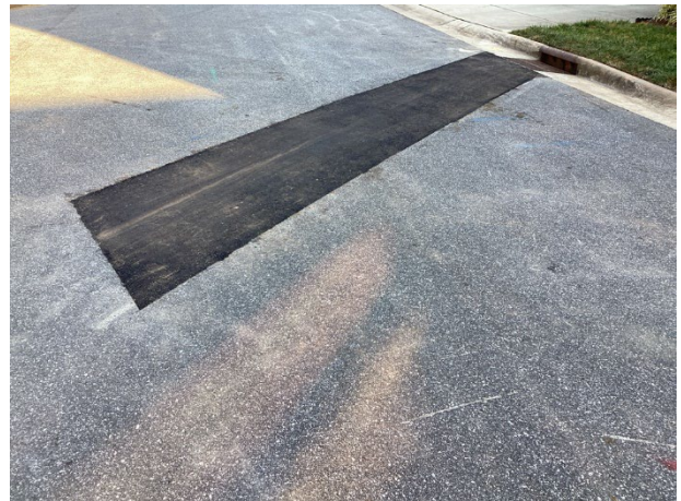
Catch basin recent repair
