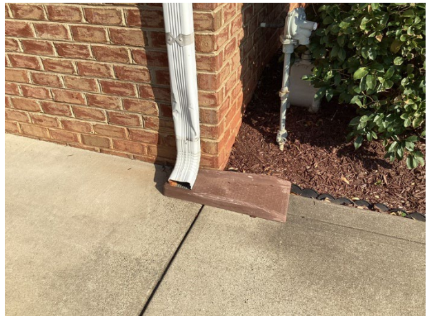
Downspout damage
