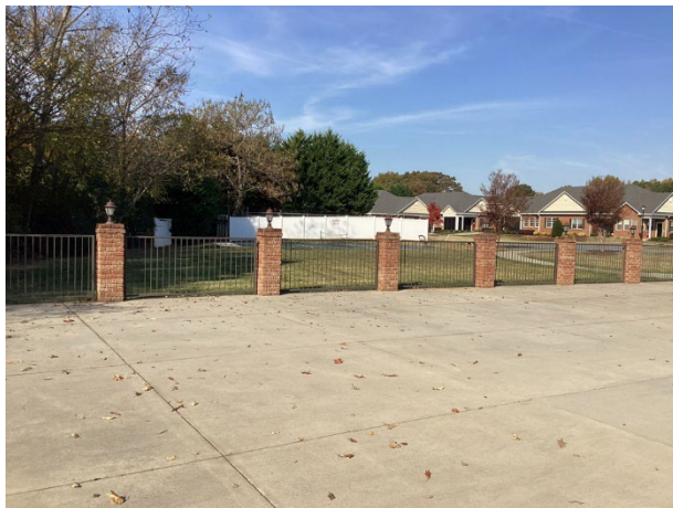
Steel pool fence overview
