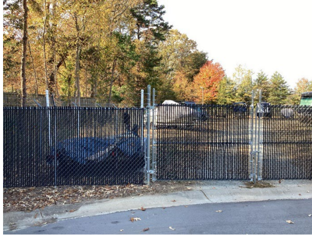
Chain link fence at boat storage
