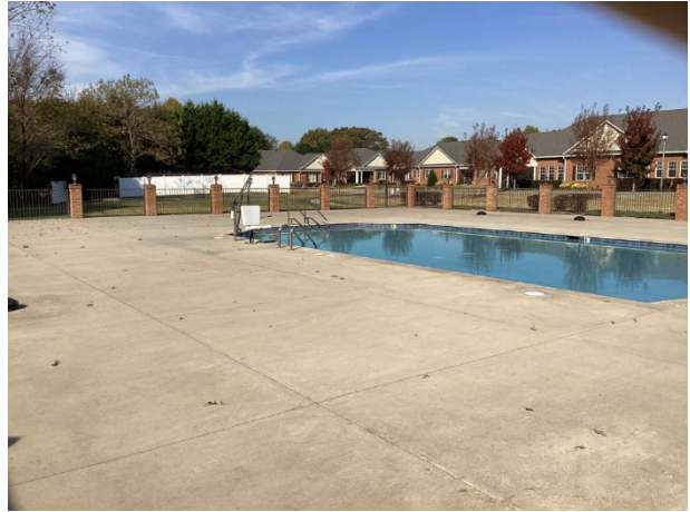
Concrete pool deck overview
