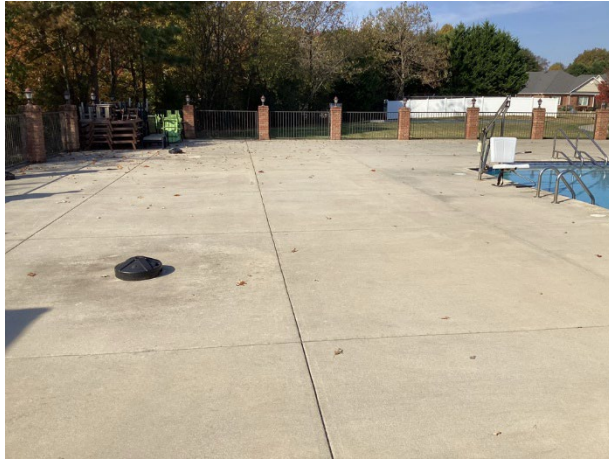
Concrete pool deck overview
