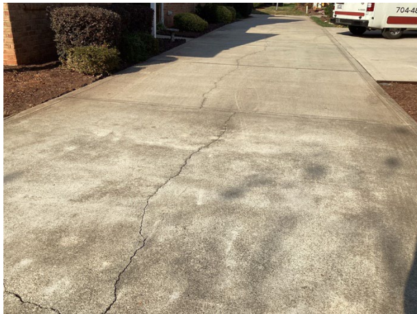
Driveway cracks
