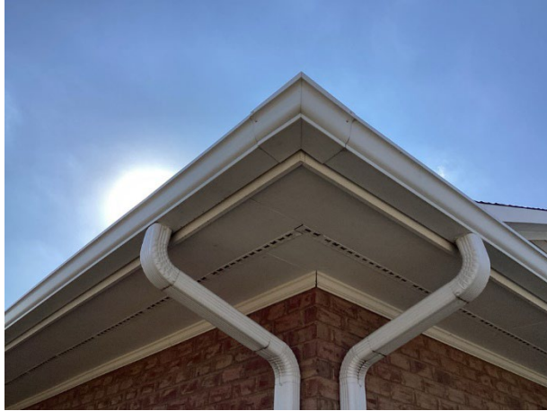
Aluminum gutters and downspouts
