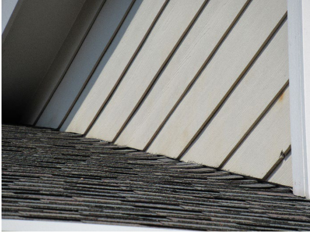
Dormer siding interface
