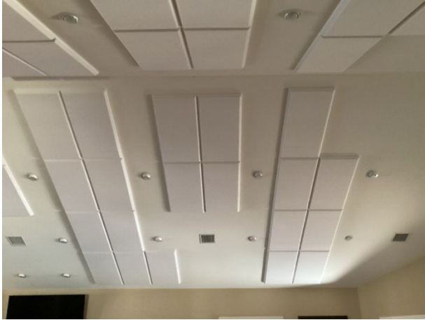
Club house Ceiling
