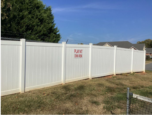
Vinyl fence at lift station
