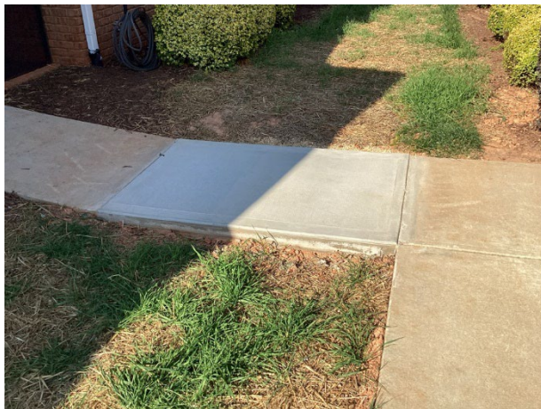
Concrete sidewalk recent repair
