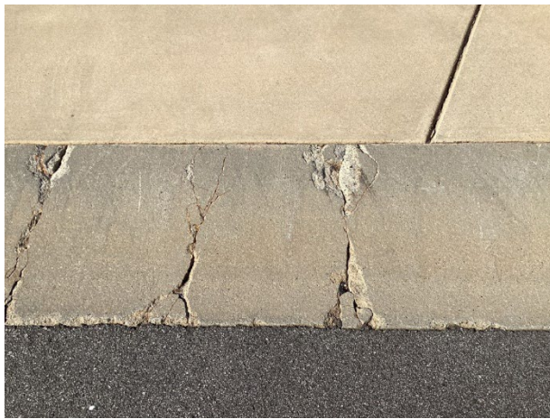
Concrete cracks
