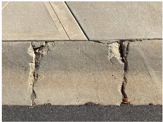
Concrete spalls
