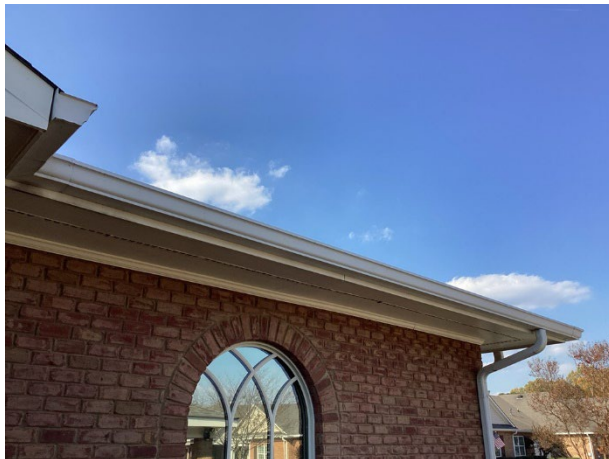
Aluminum gutters and downspouts
