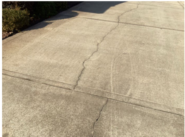
Driveway cracks
