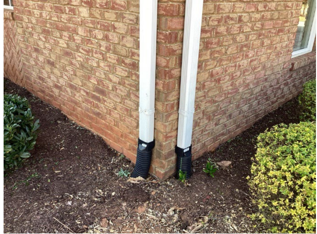
Aluminum gutters and downspouts
