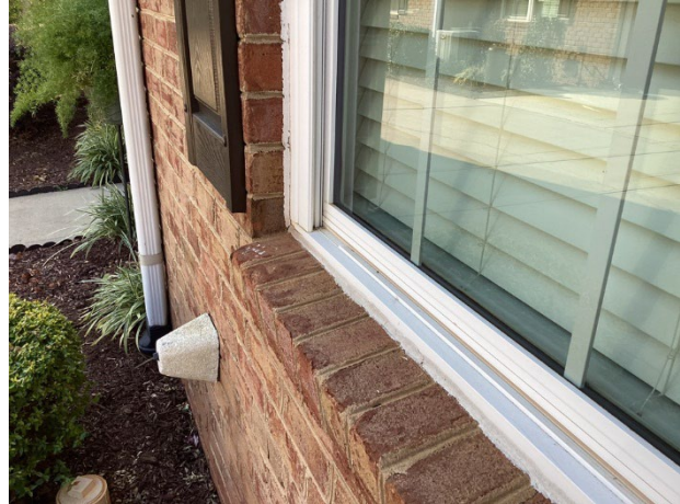
Masonry sill and sealant at window
