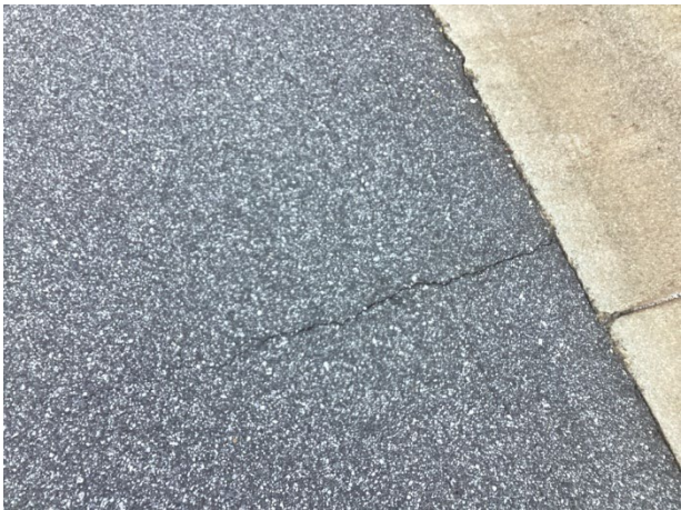
Pavement cracks
