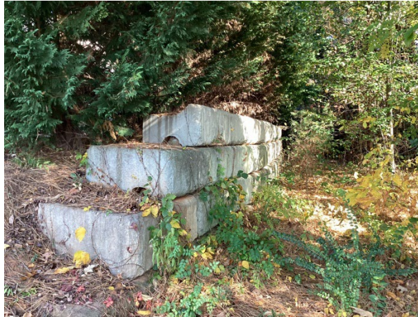
Masonry retaining wall
