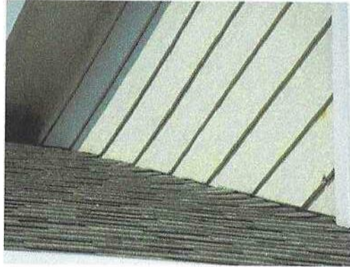
Dormer siding interface
